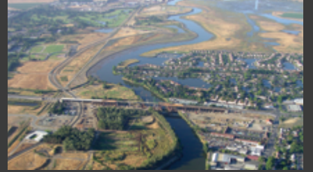
Napa River, state of the art floodplain restoration in Northern California.
