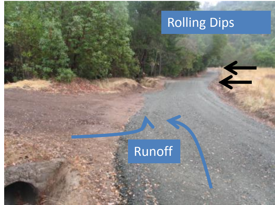
Road runoff from side road treated separately, runoff dispersed via rolling dips (away from gully and stream)
